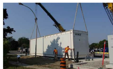
A crane moves one of the AST modules into place. Photo by: AST Modular
