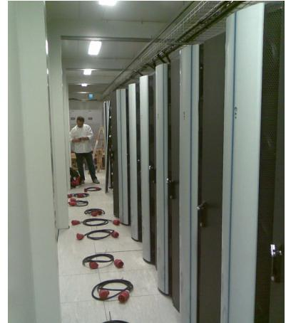
The site had to retain a small footprint whilst maximising the density and be highly efficient 340kW - for this they requested 15kW - 30kW capacity for each cabinet of the 23 cabinets, including the cooling of 6 IBM SAN cabinets using the same system. The water supply temperature of 15°C was required for the chillers and dry air cooler already chosen for the external space.
