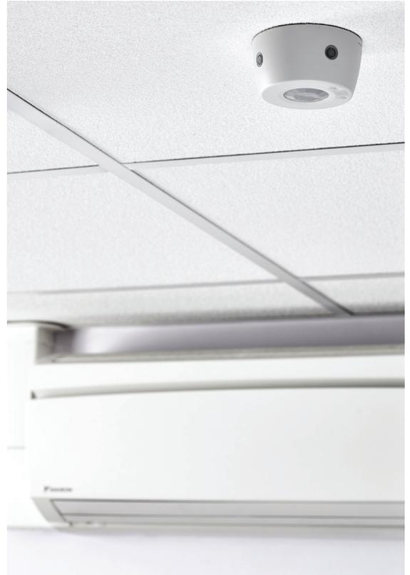
A surface mounted air conditioning (AC) controller that provides auto on/auto off switching of infrared controlled AC units, based on occupancy. As it controls use, significant energy savings can be achieved.
