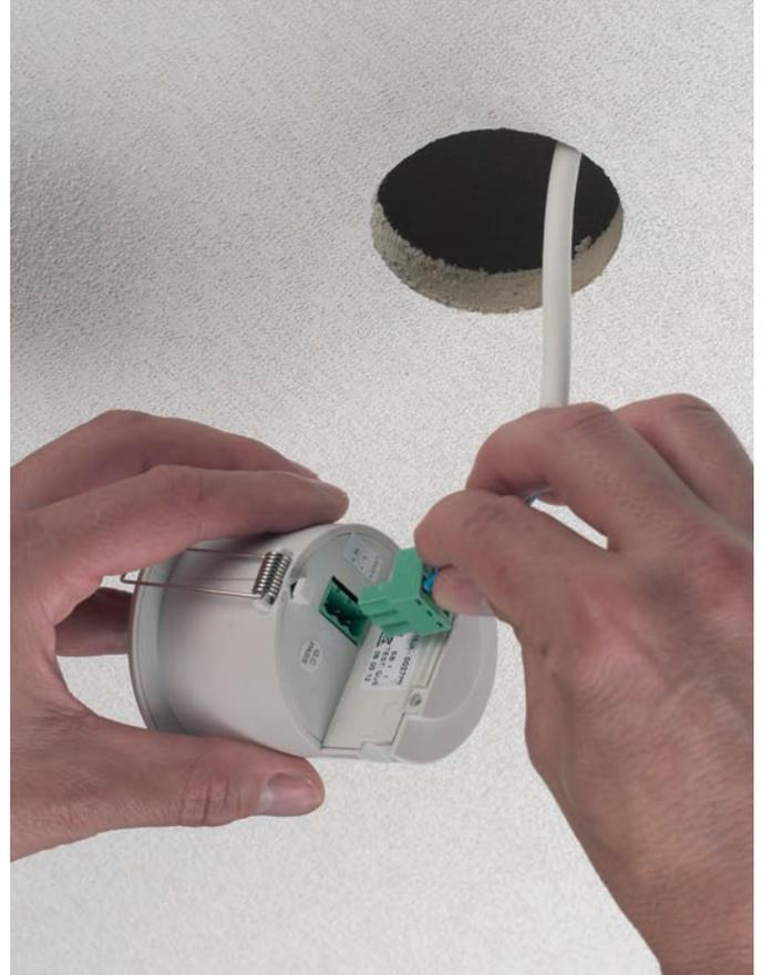
EBDSPIR-KNX is a compact PIR detector suitable to be mounted either flush or in a surface mount box. Designed with switch input connectors, the simple to install EBDSPIR-KNX is suitable for narrow ceiling voids and still offers sensitive detection.
