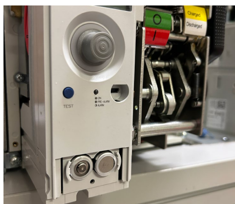
Emplacement batteries
