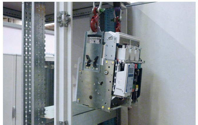
Installation of a fixed DMX-SP.
