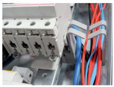
Holding vertical wiring in place
