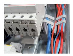
Holding vertical wiring in place
