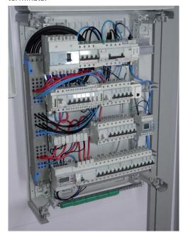
• Three-phase horizontal distribution using 125 A plug-in HX³ supply busbar with 24 modules Cat. No. 4 052 40 using accessory Cat. No. 4 052 24.
