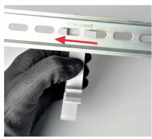
Fitting a guide ring for horizontal wiring
