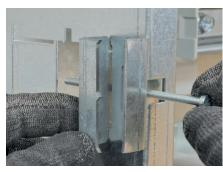
After cutting out the cable feedthroughs and positioning the enclosure, insert the mounting lugs and tighten them
