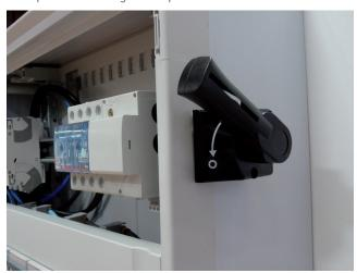
A template is provided with the side/front handle for drilling the side panel
