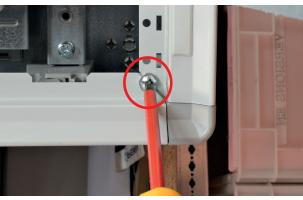
Remove all 4 screws (one in each corner: see photo) and take off the top, bottom, left- and right-hand panels
