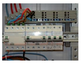
$\bullet$  Three-phase horizontal distribution using 125 A plug-in HX³ supply busbar with 24 modules Cat. No. 4 052 40 using accessory Cat. No. 4 052 24.
