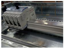
Mounting with a plate and the rail height spacer next to it
