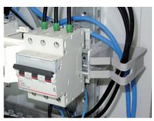
Holding vertical wiring in place
