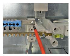
The support integrated at the back of the cabinet is used to fix the bars both horizontally and vertically
