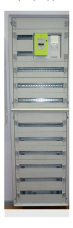
Set of 2 joined cabinets, with meter and incoming circuit breaker at the supply end
