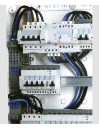
Do not work on the 4-pole vertical supply busbar when it is live.
