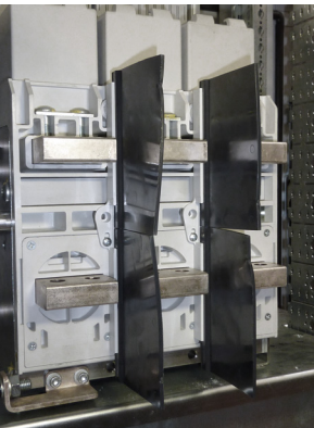
Insulated shields mounted on the fixed DMX 3 3P
