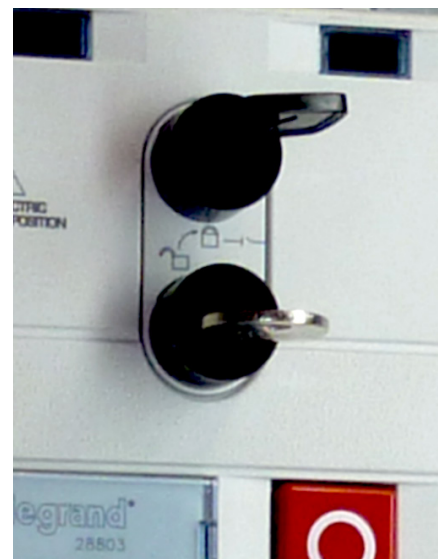
Locking accessory equipped with two cylinders of different types
