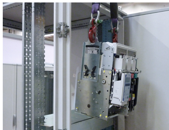
Placement of a fixed DMX 3
