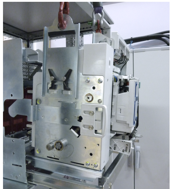
Placement of a draw-out DMX 3 in its base
