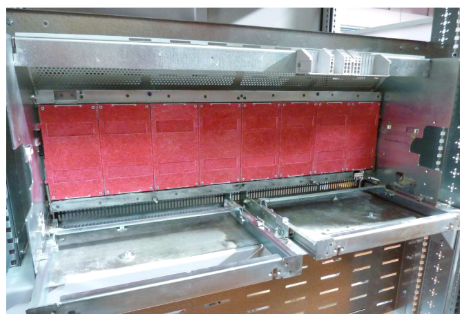
Empty base for DMX 3 - Size 6300 - 4-pole - Cat.No 0 289 14 and terminal block Cat. No. 0 290 12
