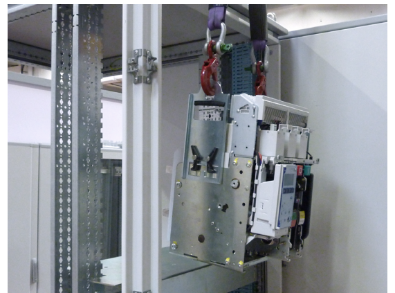
Placement of a fixed DMX 3
