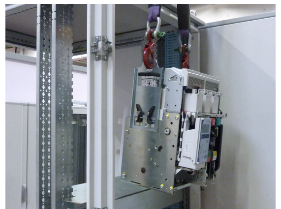
Placement of a fixed DMX 3
