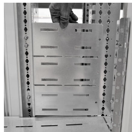
The spare compartments guarantee 3b form, required for IS 223, 233 and 333.
