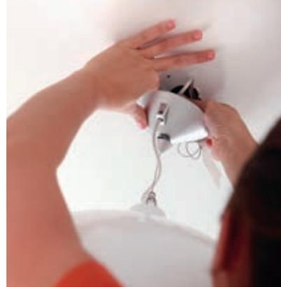
LES BOÎTES DES POINTS DE CENTRE DOIVENT ÊTRE ACCROCHÉES À LA STRUCTURE DU BÂTIMENT PAR UNE TIGE FILETÉE, UN CÂBLE...
